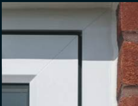
Standard - Corners welded (sash and outerframe)
